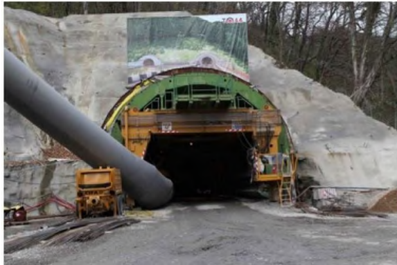
Pic. 3 Tunnel N°1
